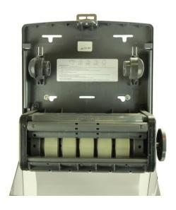
Step 2: Insert jumbo paper towel roll (maximum diameter 8"). Ensure roll hangs "under" as per photo
